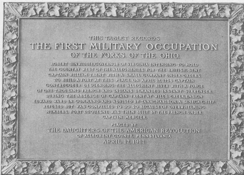
MARKER PLACED ON THE SITE OF FORT PITT, PA.
